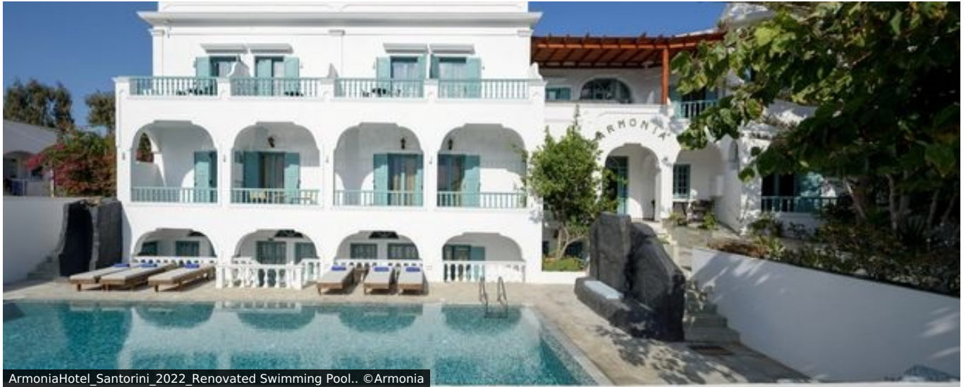
ArmoniaHotel_Santorini_2022_Renovated Swimming Pool.. ©Armonia
